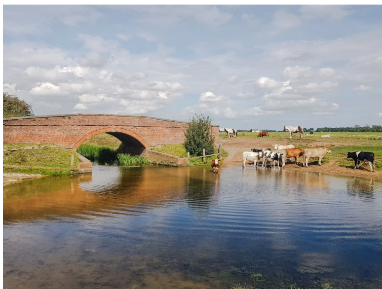
Brickie Bridge on Swinemoor
