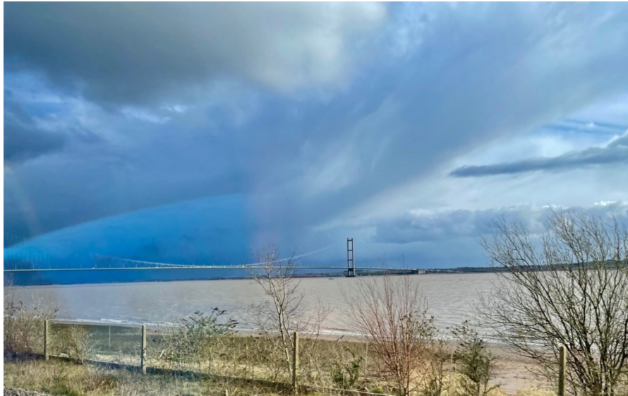
March weather over the Humber Bridge - Dick Lidwell
